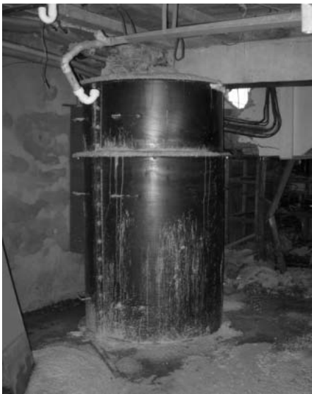
Damaged columns with completed encasement 4-9
