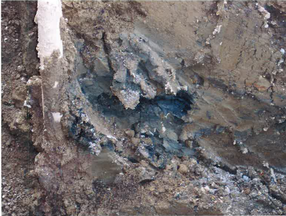
Photo 5: Southerly view of the impacted soil seam along the south wall of the excavation prior to its removal.
