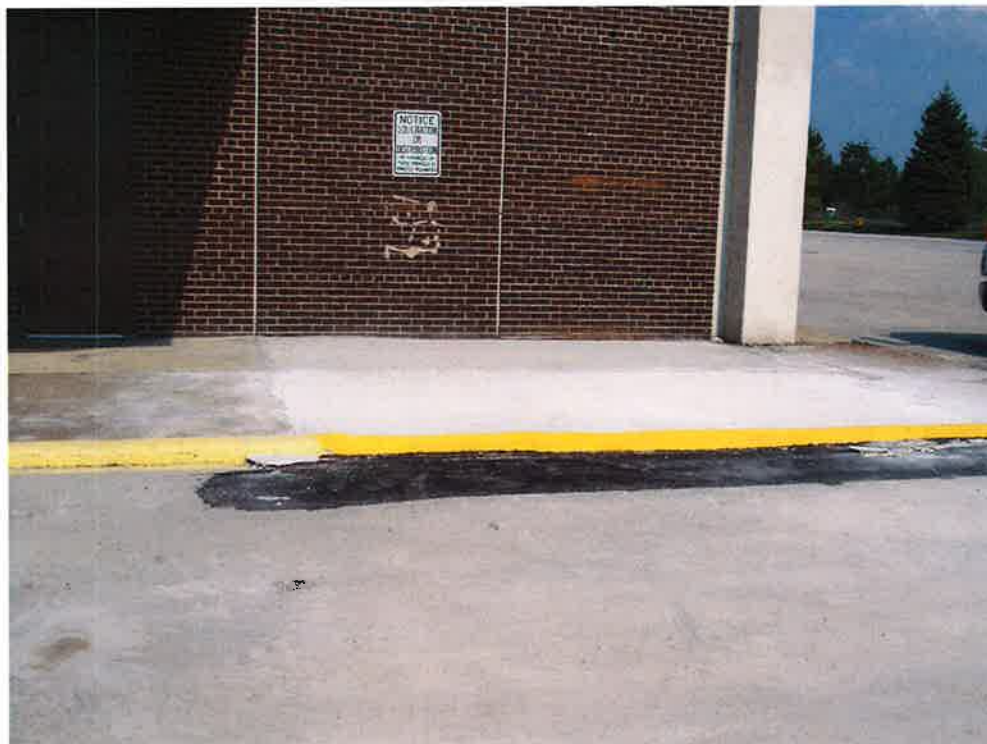
Photo 8: Looking easterly at the completed excavation and restored concrete and asphalt.
