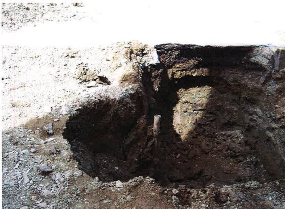
Photo 6: Westerly view of the excavation. Note the pea gravel cave-in (bottom left) from the former UST cavity.
