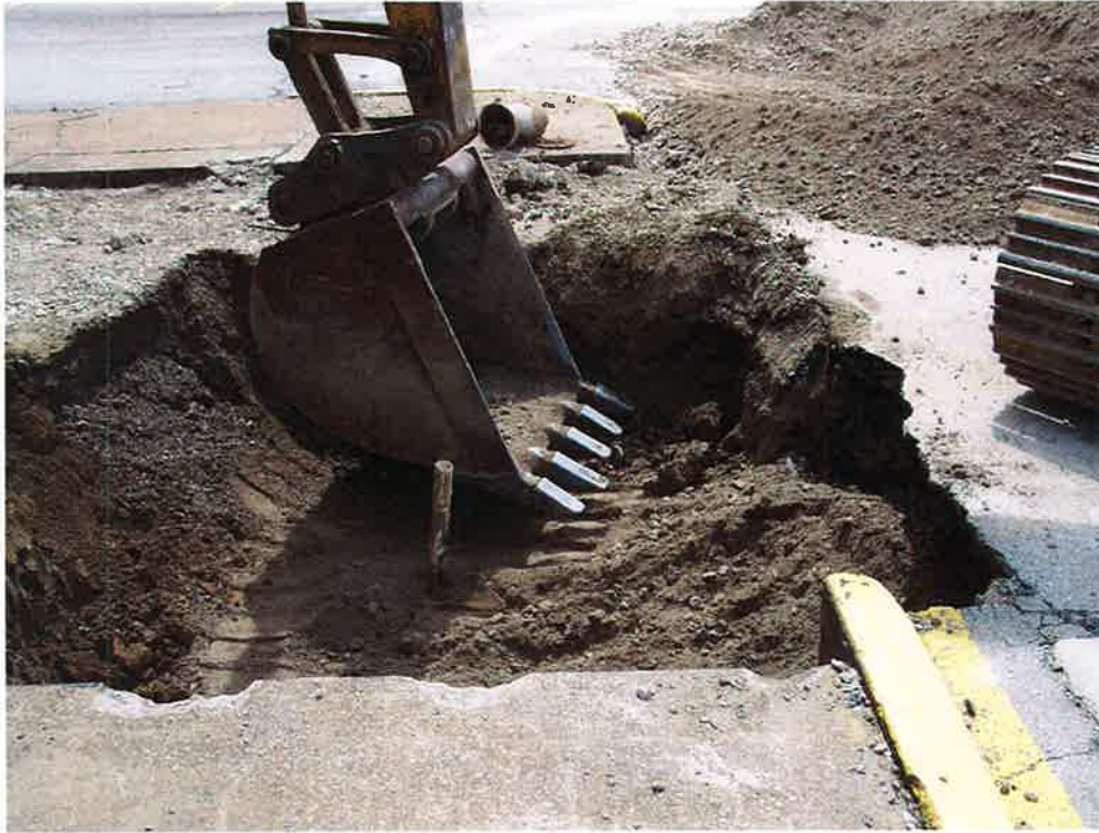
Photo 7: View of the excavation during backfilling activities. MW-1 and MW-2 (bottom right of photograph) were cut three feet below grade and sealed.
