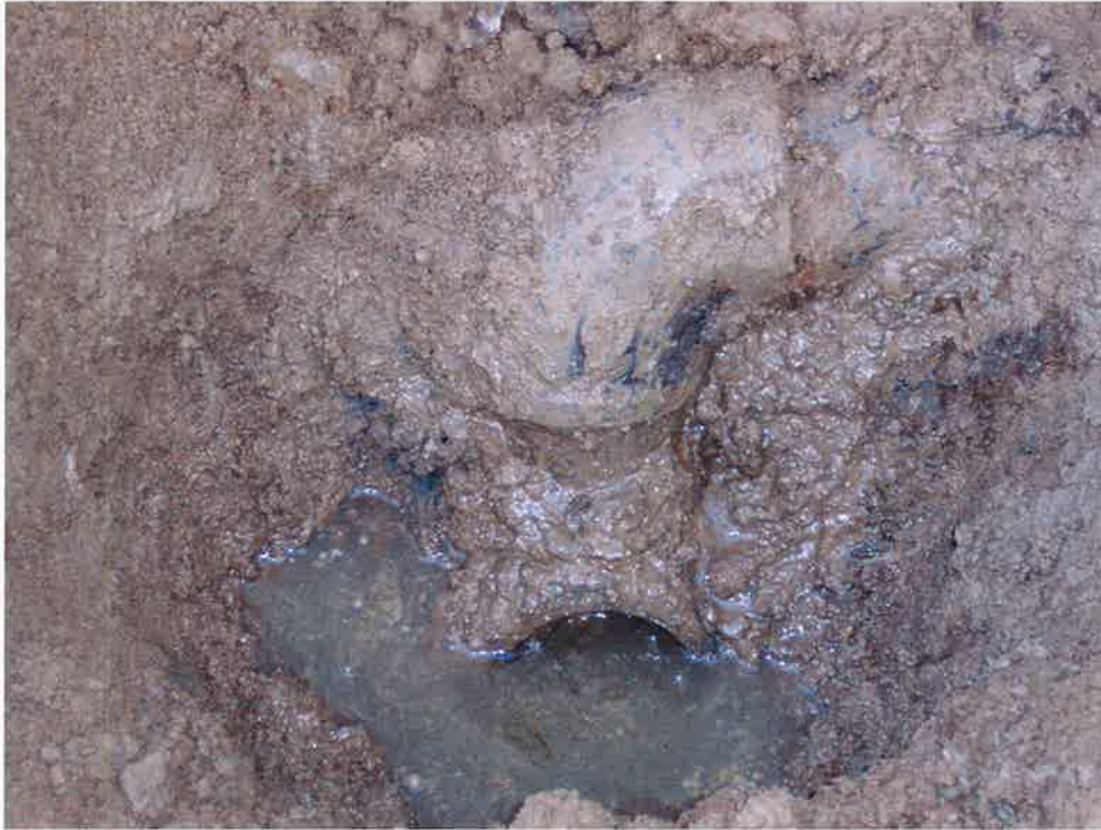
Photo 3: View of the abandoned pipe from the former used oil UST. This pipe was removed prior to backfilling the excavation.
