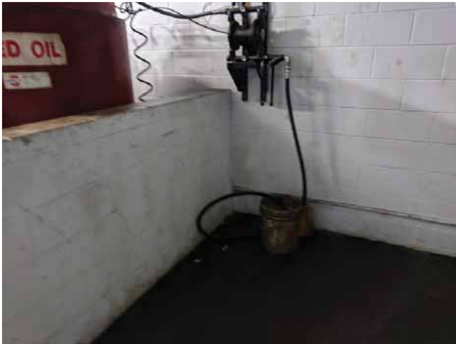
Photo 54: View of oil staining on the concrete outside of the AST containment area.
