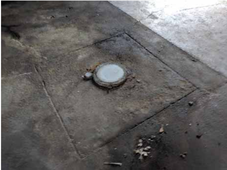
Photo 44: View of an underground hydraulic lift filled with concrete.
