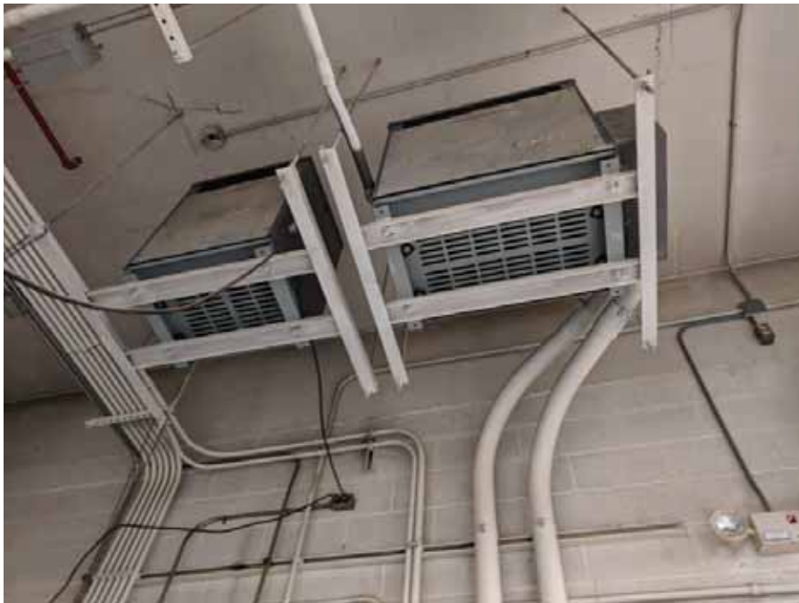
Photo 18: View of two dry-type transformers located within the mechanical room on the second floor of the Sears store.
