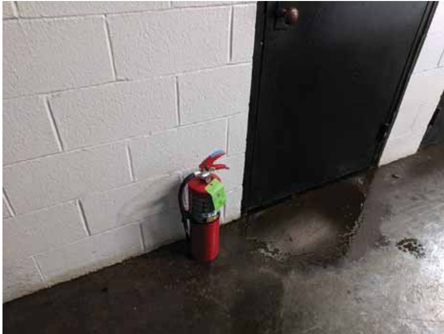
Photo 57: View of hydraulic oil seeping out of the door of the elevator equipment room.
