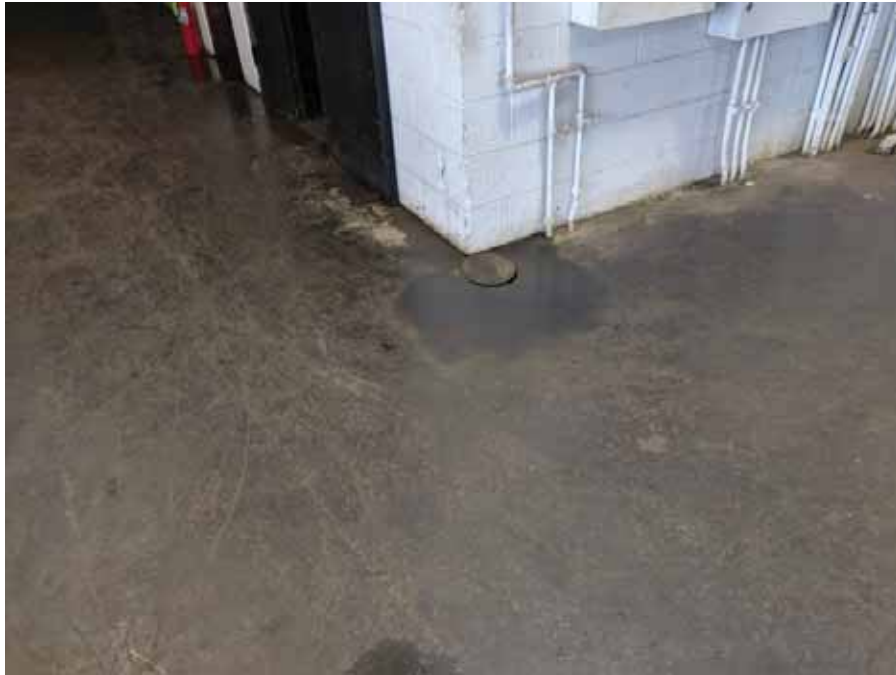
Photo 59: View of a drain that has oil staining around it located within the Sears Auto Center.
