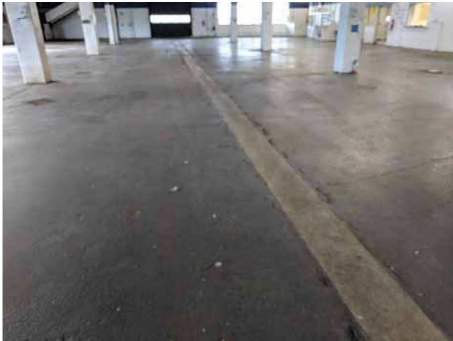
Photo 70: View of a former trench drain located on the first floor of the Sears Auto Center.
