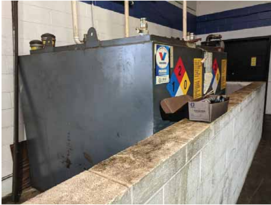
Photo 51: View of the two new oil ASTs located within the Sears Auto Center.
