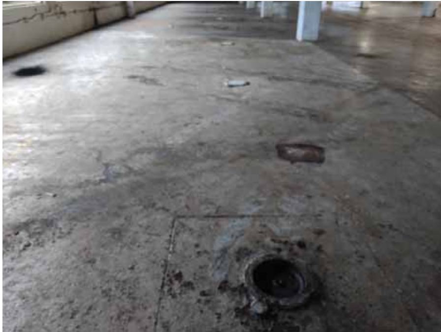
Photo 45: View of the underground hydraulic lifts (most filed with concrete) located within the Sears Auto Center.
