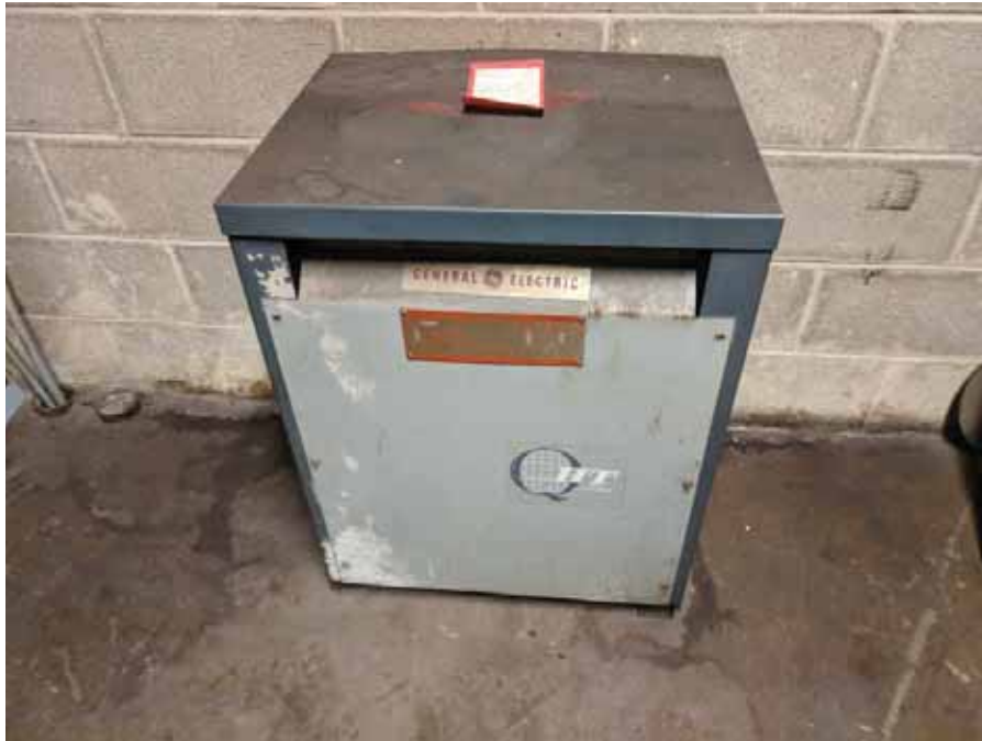
Photo 67: View of a dry-type transformer located in the mechanical room on the second floor of the Sears Auto Center.
