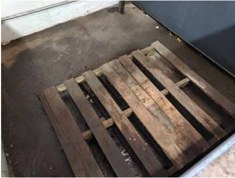
Photo 53: View of oil staining located on the concrete containment area beneath the ASTs.
