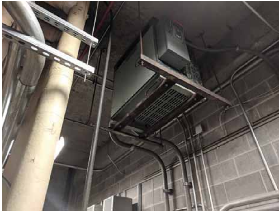
Photo 11: View of a dry-type transformer located in mechanical room on the roof of the Sears store.
