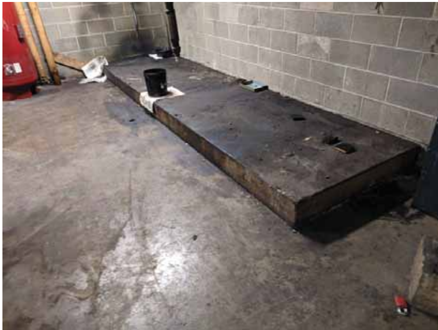
Photo 66: View of oil staining on the concrete in the second floor mechanical room of the Sears Auto Center.
