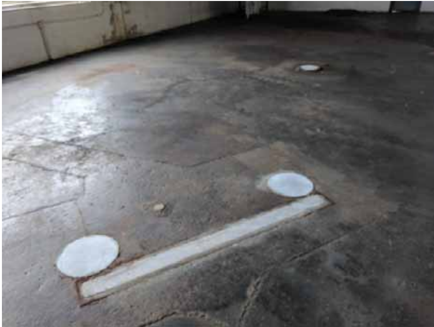
Photo 47: View of underground hydraulic lifts filled with concrete within the Sears Auto Center.
