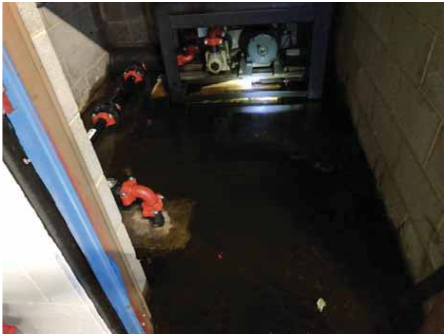
Photo 56: View of hydraulic oil located on the concrete floor of the elevator equipment room.
