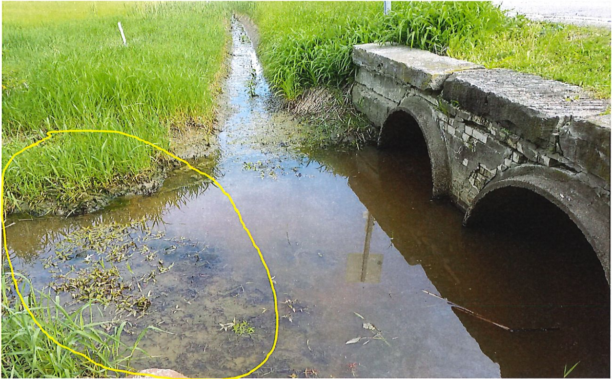
Figure 9- Built up sedimentation at exit of culverts and roadside lateral from North Ridgeville.
