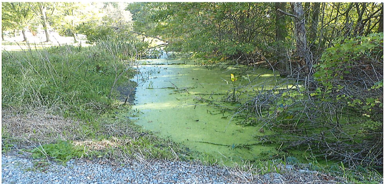
Figure 9- Ditch has become shallow with little shape and no flow.
