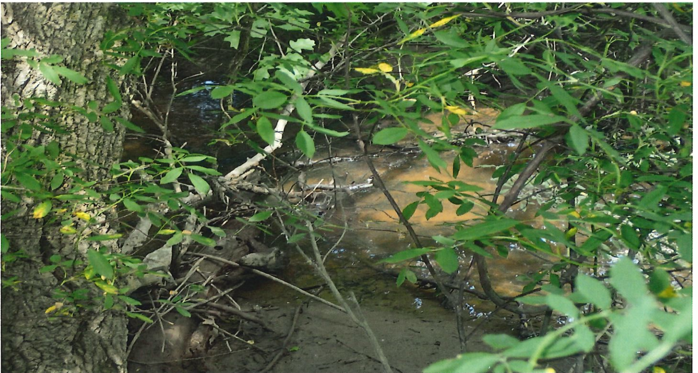
Figure 3- Sticks, debris, and silt obstructing flow
