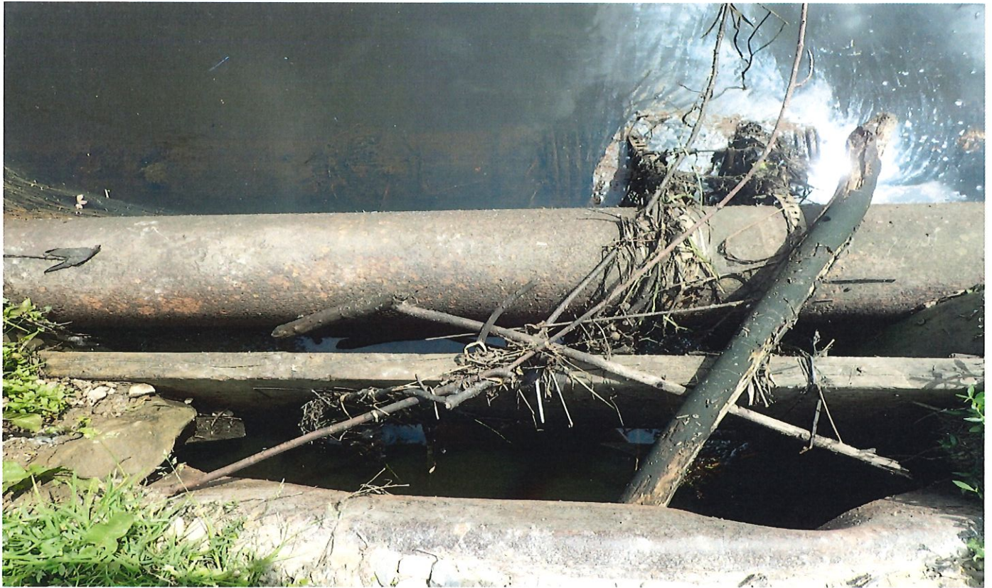
Figure 10- Pipe and board obstruction attached to culvert
