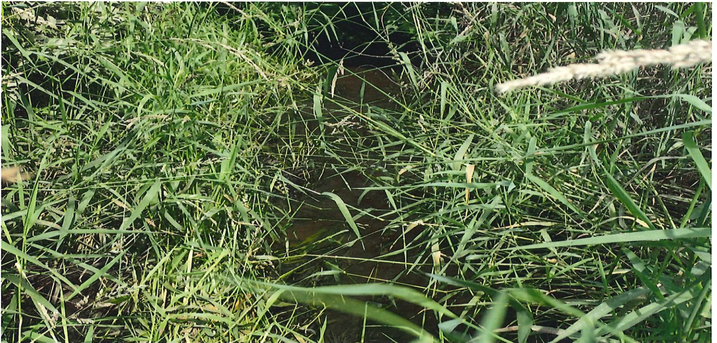
Figure 11- Ditch has significant silt build up in some stretches causing narrowing and pinch points.
