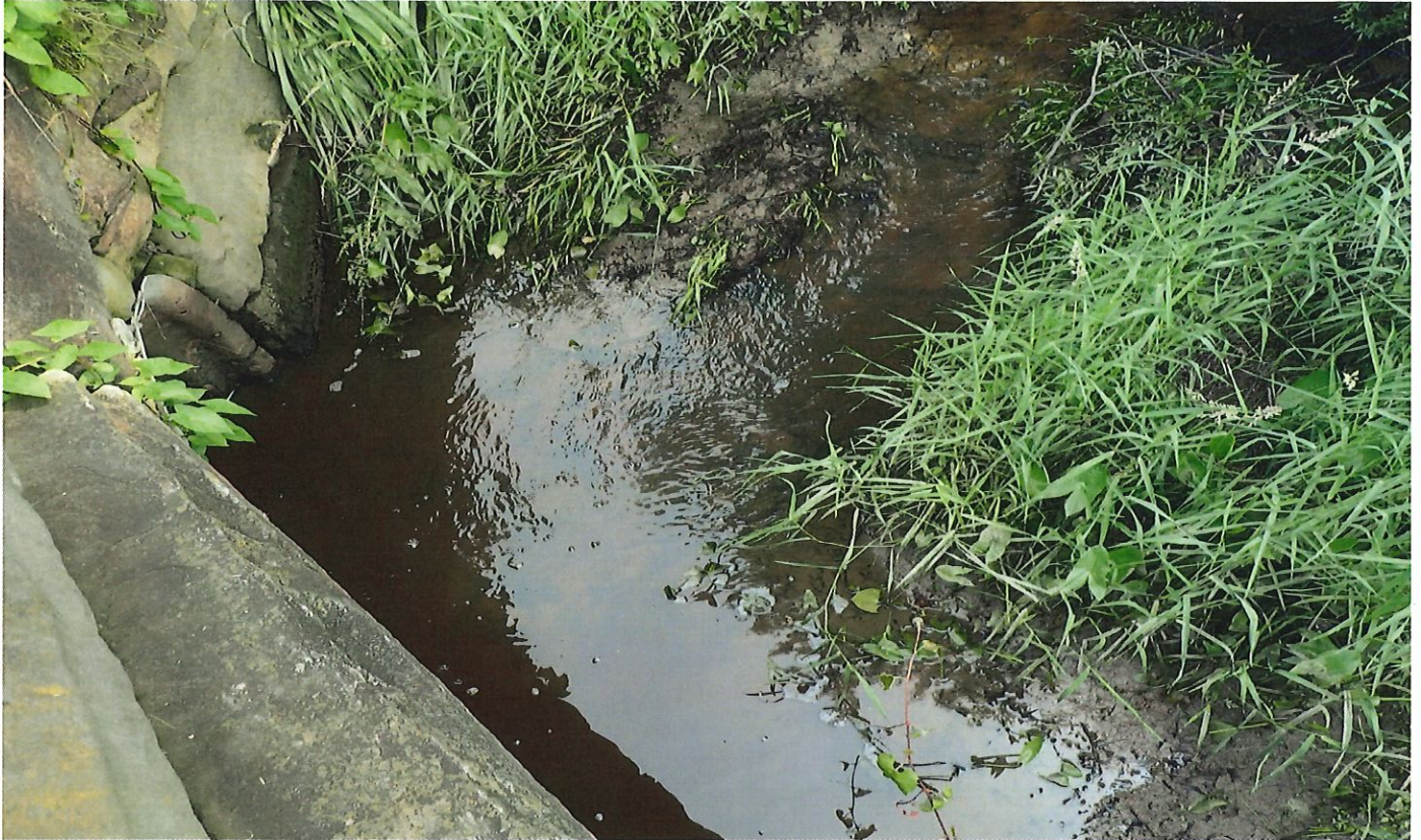
Figure 2- Culvert under Reed Rd. Silt Built up on sides and vegetation overgrowth causing narrow pinch point.
