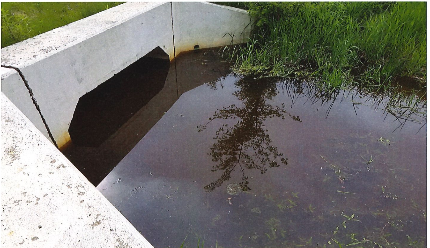
Figure 4- Large box culverts with 24"+ of ponding water
