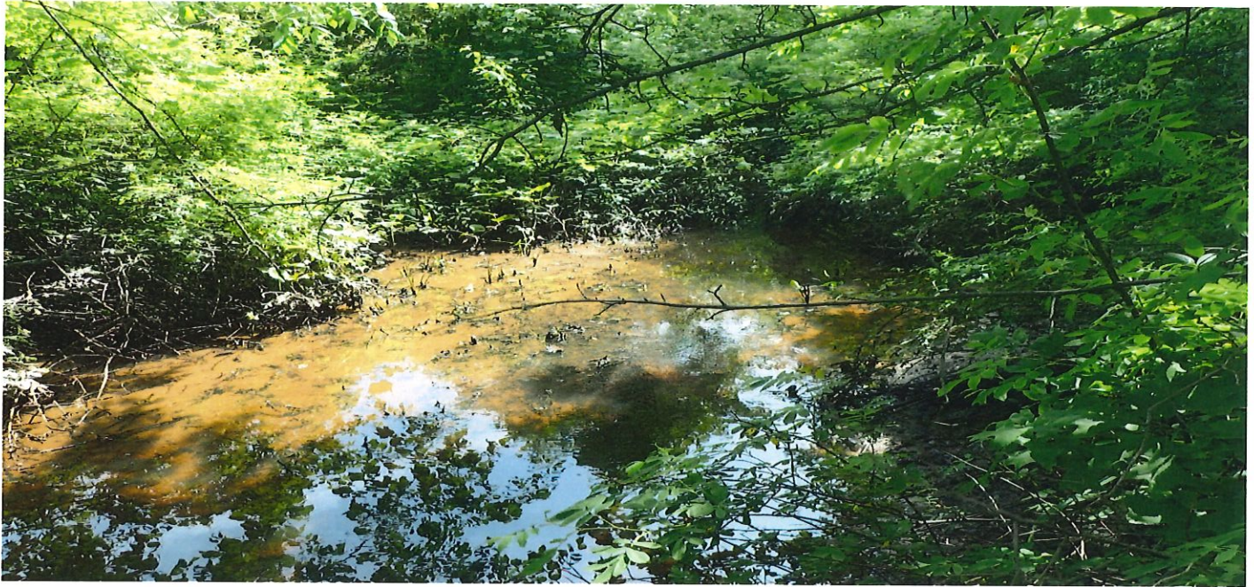
Figure 12- Some stretches are wide and flat but a very thick silt layer has developed causing ponding of water only inches deep over wide areas. Almost as if the ditch has become non-existent in some areas.
