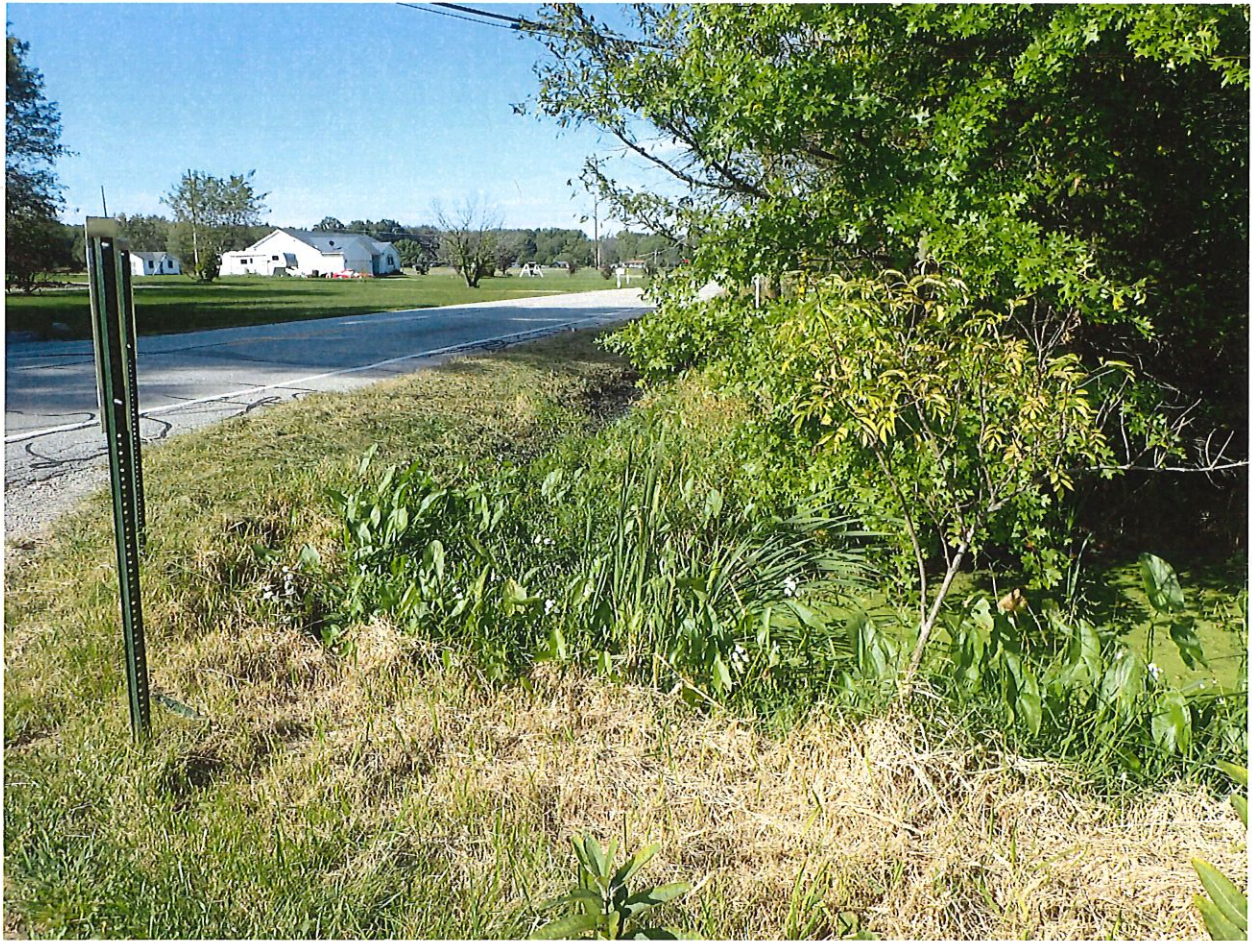
Figure 8- Roadside ditch could be regraded and cleaned of sediment to allow water to flow. It sits like swamp currently growing duck weed and has become anoxic.
