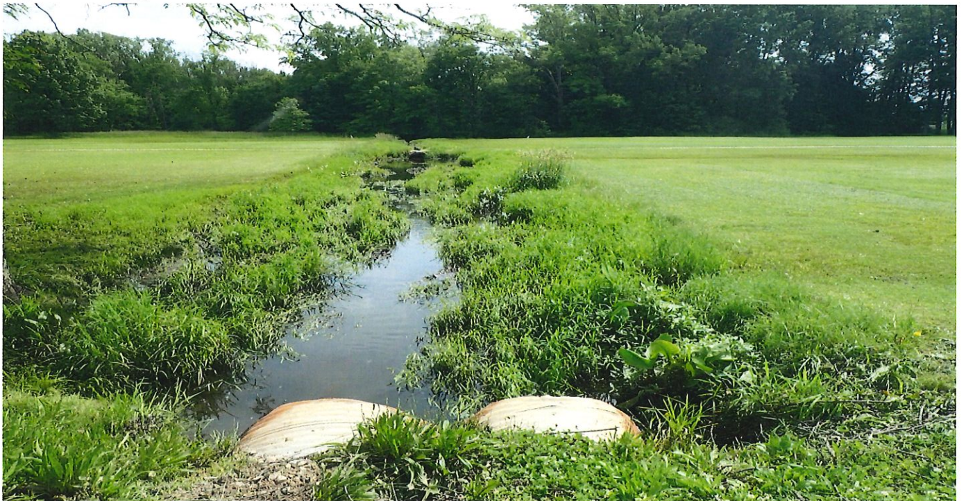
Figure 9- Creek Wood Golf Course cart paths. One path has two approximately 36" culverts, one with lots of siltation. The other path has one approximately 36" culvert with a piece of board and other obstructions attached (Fig 10)
