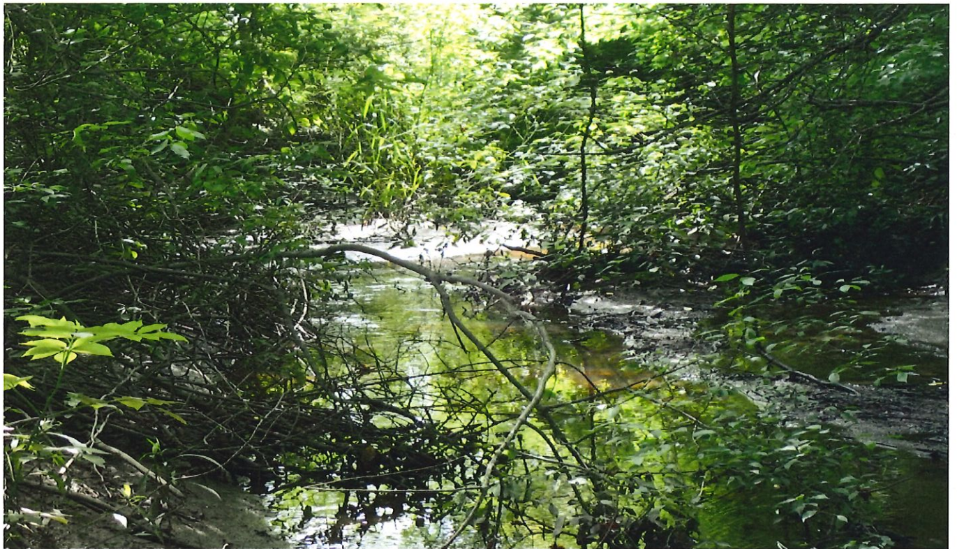
Figure 5- Silt built up in ditch causing sluggish flow.
